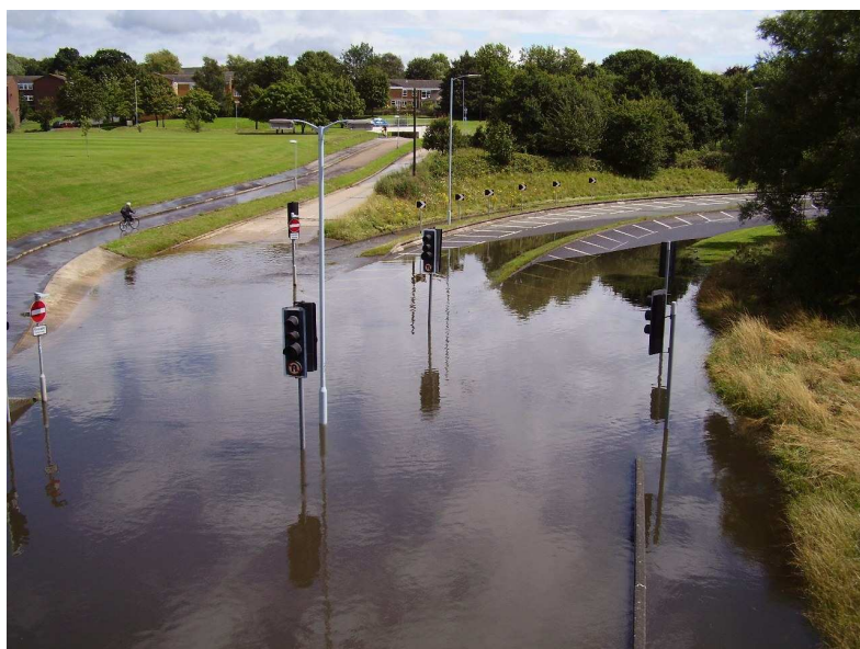
Figure 3.5.6: Photograph of Ellesfield Avenue near Mill Pond, July 2007
